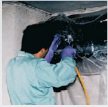
Cleaning fins of A/C unit.
