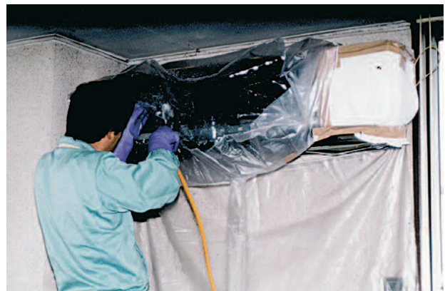
Cleaning fins of A/C unit.
